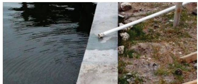
Illegal dewatering to surface waters
