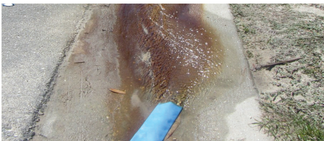
Illegal dewatering to the stormwater system
